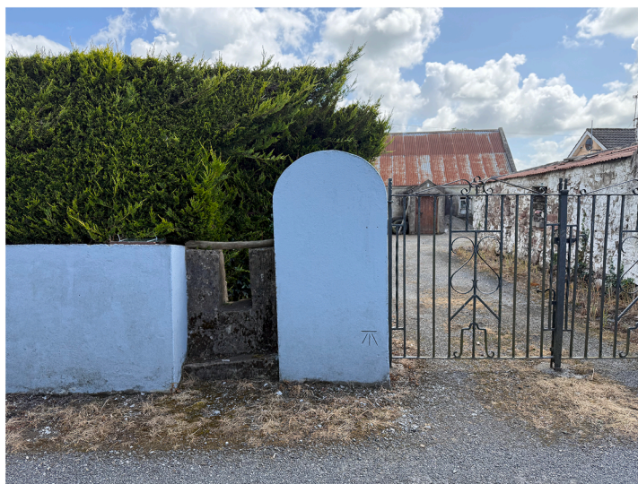
Fig. 5. An example of a modern interpretation of a bench mark, the original of which is lost to renovation at the same site.
