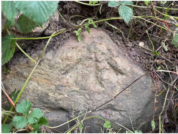
Fig. 6. An example of a 'pivot' bench mark revealed from hedging on a road side near Bilboa in the townland of Clooteen. The contextual image also shows the extent of overgrowth on a typical roadside dry stone wall whereby 37 % of bench marks are classed as 'Lost to nature'.
