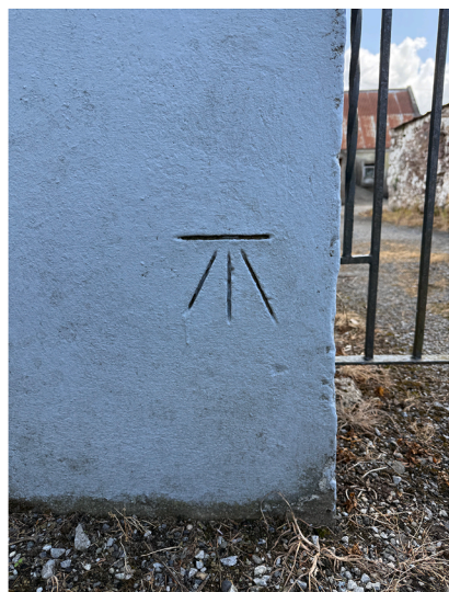
Fig. 5. An example of a modern interpretation of a bench mark, the original of which is lost to renovation at the same site.
