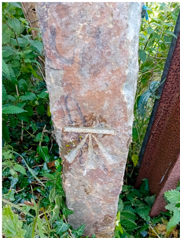
Fig. 4. An example of a 'cut' bench mark chiselled into an upright sandstone pillar (gate post), in Coole East townland, south west of Athea.
